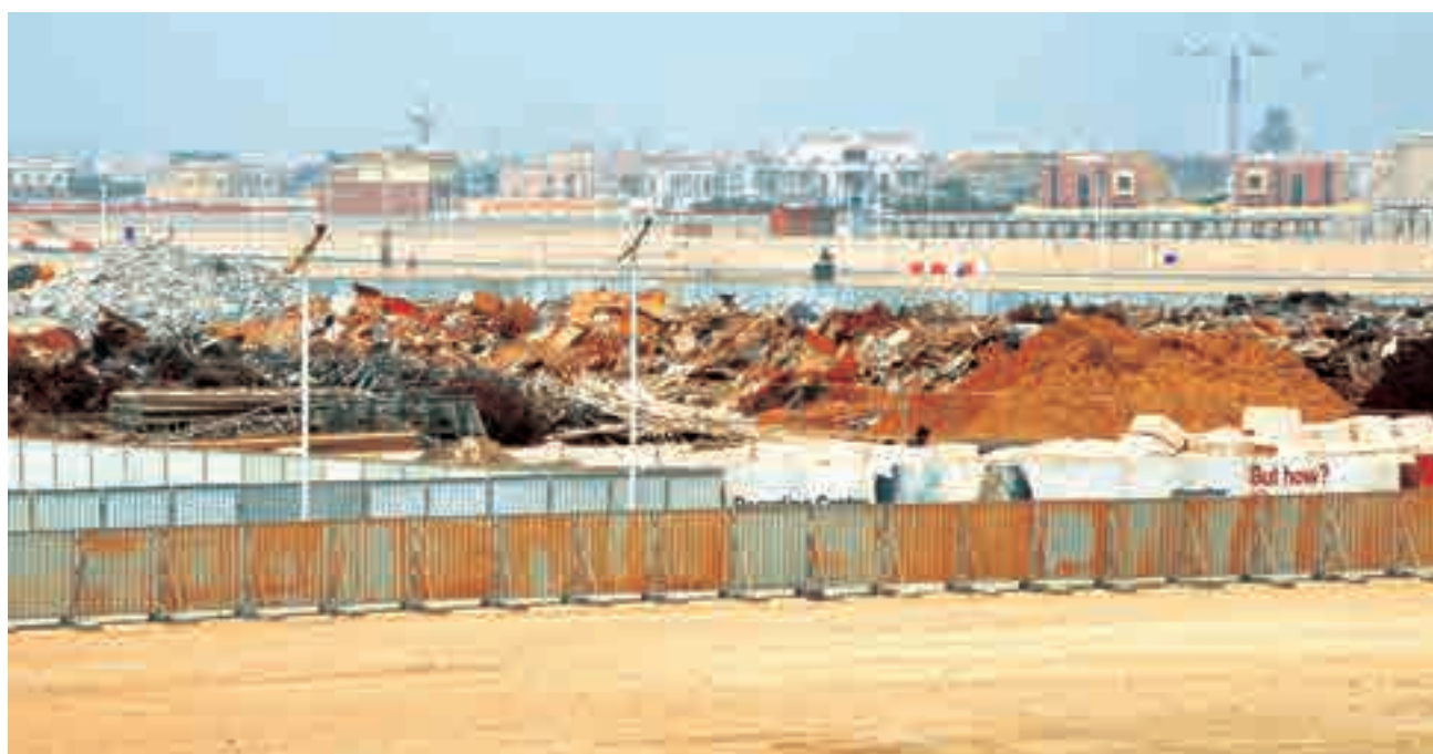
Bottom: Construction solid waste (Courtesy: EAD)
